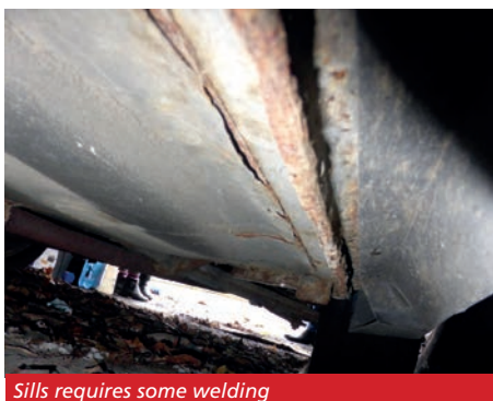
Sills requires some welding
